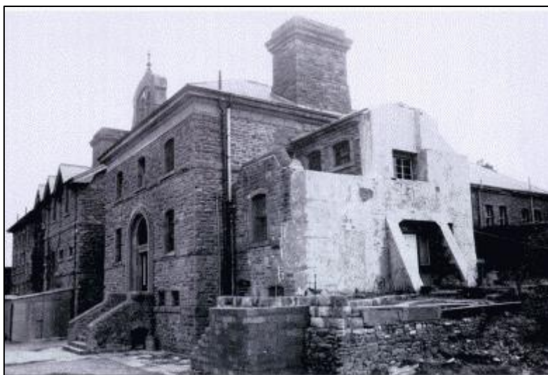
Brecon County Gaol 7
